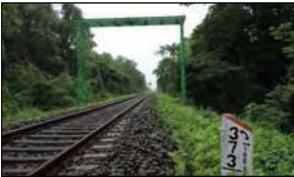
Figure 17.2c. Iron bridge constructed over the train track in Hoollongapar Gibbon Sanctuary to serve as a canopy bridge for movement of hoolock Gibbons. Photo credit: Sonali Ghosh
