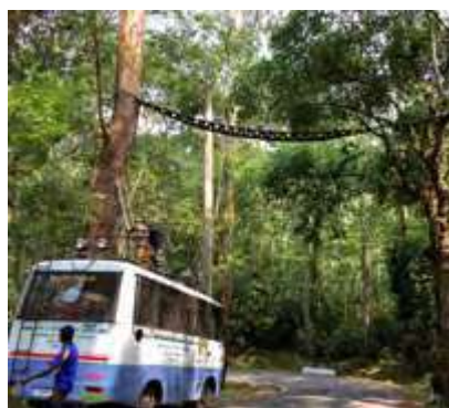
17b Canopy bridge connected to the trees on both sides of the Highway. Photo credit: Ganesh Raghunathan
