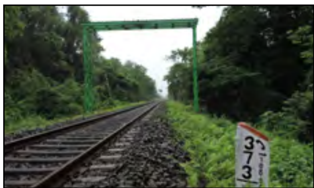
Figure 17.2c. Iron bridge constructed over the train track in Hoollongapar Gibbon Sanctuary to serve as a canopy bridge for movement of hoolock Gibbons. Photo credit: Sonali Ghosh
