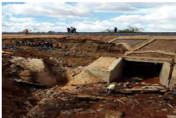
Figure 12.9 (a) Cracks in Kathekani Secondary school from construction; (b) collapse of SGR embankment due to heavy rains in Makeni. Construction blocked several rivers, formed gullies, increased flooding and destroyed roads from rising surface runoff (e.g. Kawese River in Makeni county, Darajani water pan in Mito Andei, Kibwezi East, Emali town, Mang'elele wetland, Kiboko spring); (c) Mang'elele quarry sites left unrehabilitated; (d) farmlands lost from the dumping of waste, and mango and banana trees and beehives severely affected by dust at the Mang'elele quarry site area.
